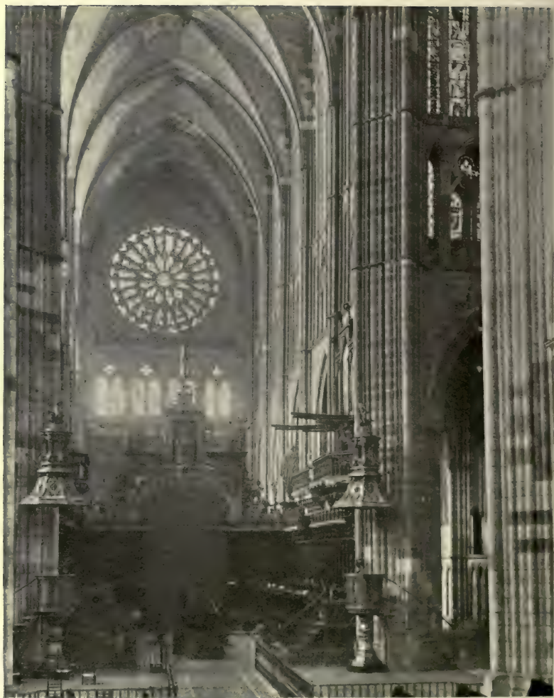
NAVE, LOOKING WEST Cathedral, Leon
